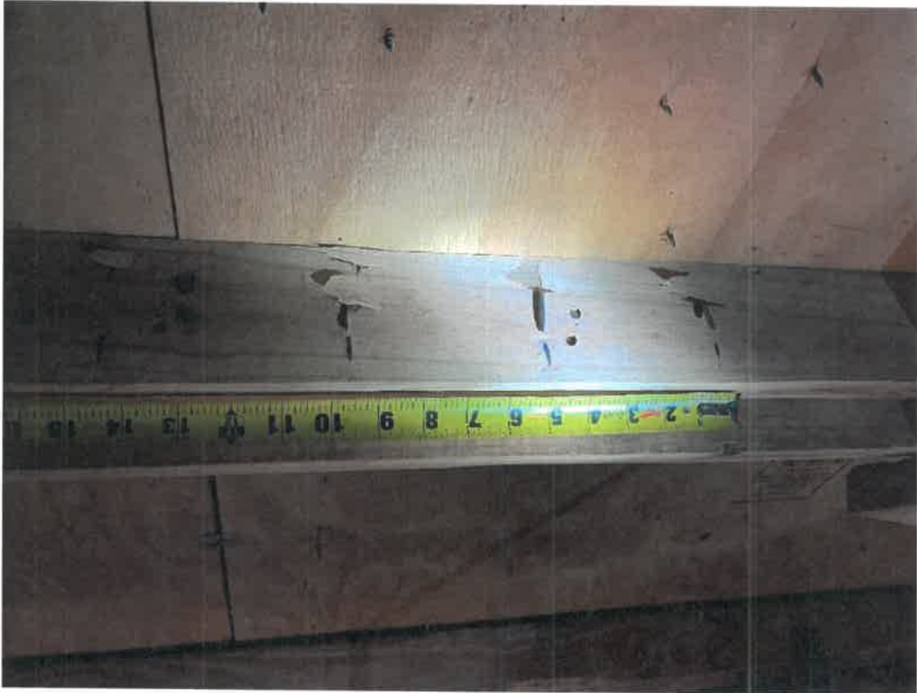
Figure 2 – Plywood Sheathing Nail Spacing (Typical)
