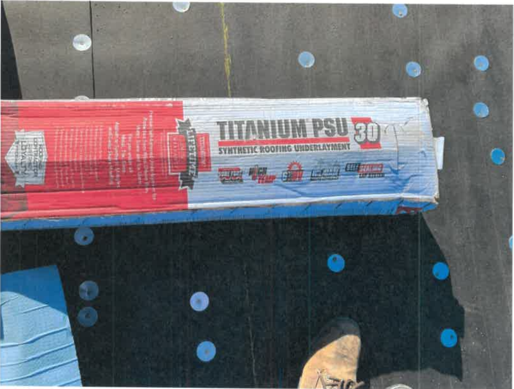
Figure 4 – Secondary Water Barrier at Sloped Section (Typical)
